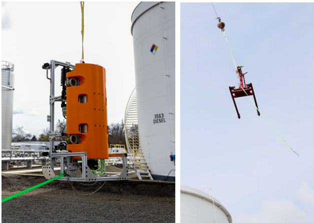
① Lift hoist and robot to tank top with small crane or boom truck
